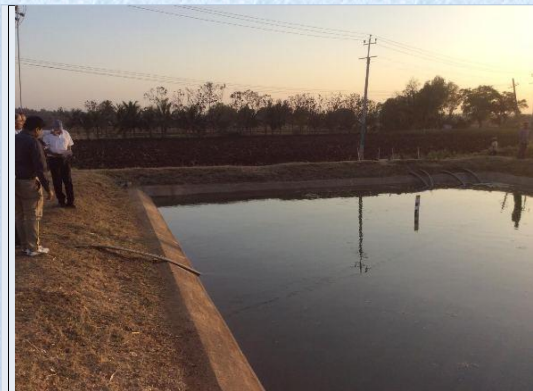
Farm Pond for Water Distribution at Field of Shiggaon Lift Irrigation Project
