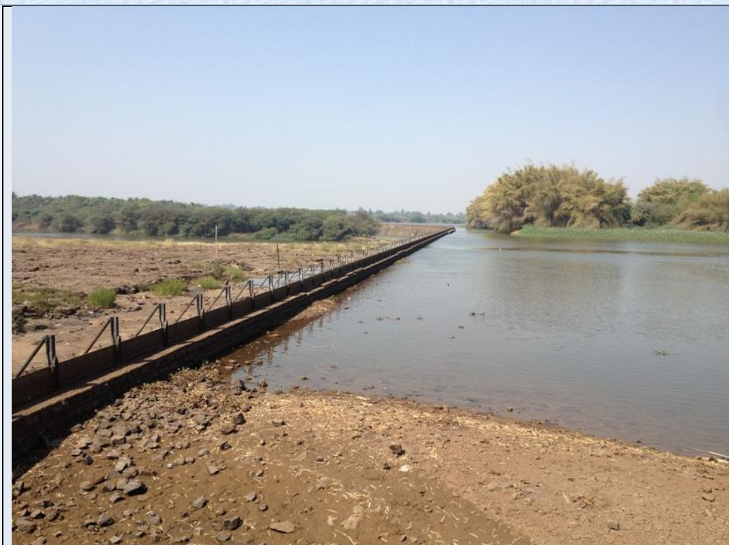
Dhupdal Weir on Ghatprabha River
