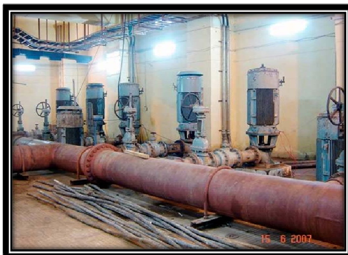
Machine Hall D & D Pumps
