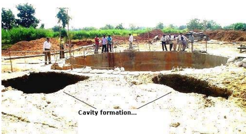
Figure: Cavity formation at @ RD 17212.921m
