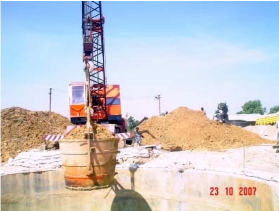
Excavation from Shaft of Tunnel
