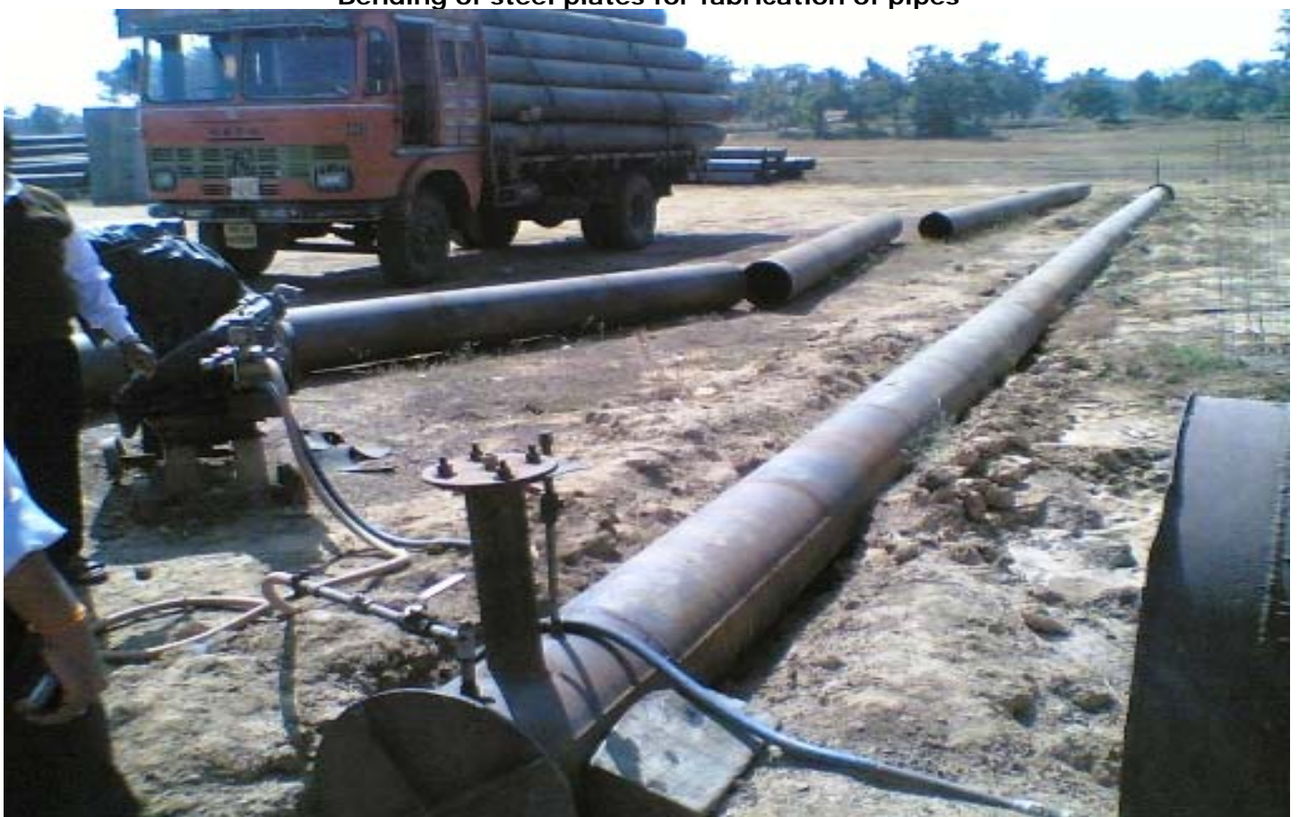
Water Proof testing for small diameter pipes
